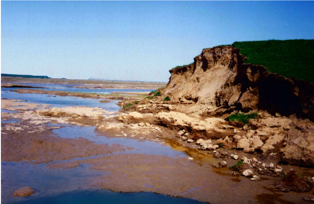
Figure 3. Dike brake at Tipari
